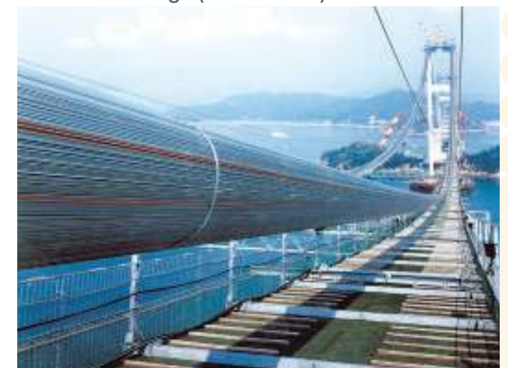
Kurushima Bridge (main cables)
