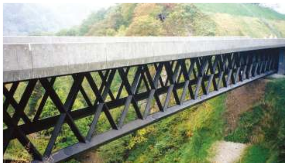
Example of a truss bridge employing square steel tubes with bent sections (Takishita Bridge, Hokkaido)
