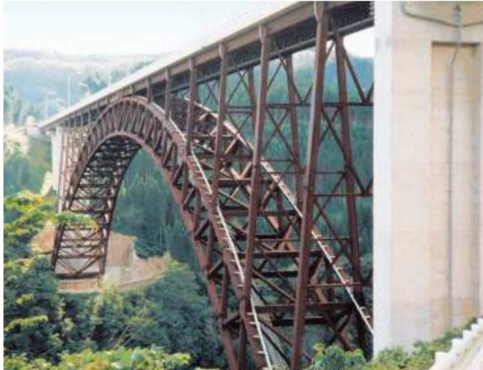
Unpainted Weathering Steel in Bridge Structure (Japan)
