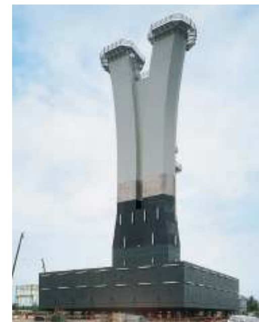
Example of a steel pier partially covered with titanium clad steel in the splash and tidal zone
