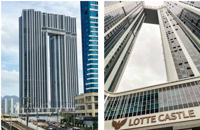
Photo 5 Exterior views of the “Busan North Port Tower”
