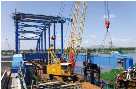
Erection of Freedom Bridge with the main span composed of Langer bridge
