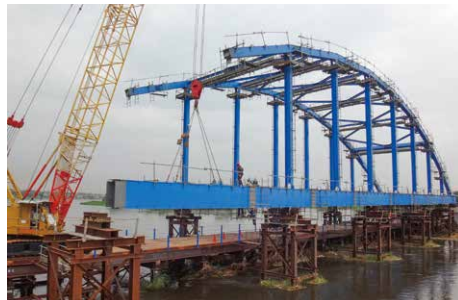
Erection of Freedom Bridge with the main span composed of Langer bridge
