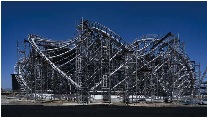
“Skew arch senbon-goshi lattice” (steel-frame erection underway)
