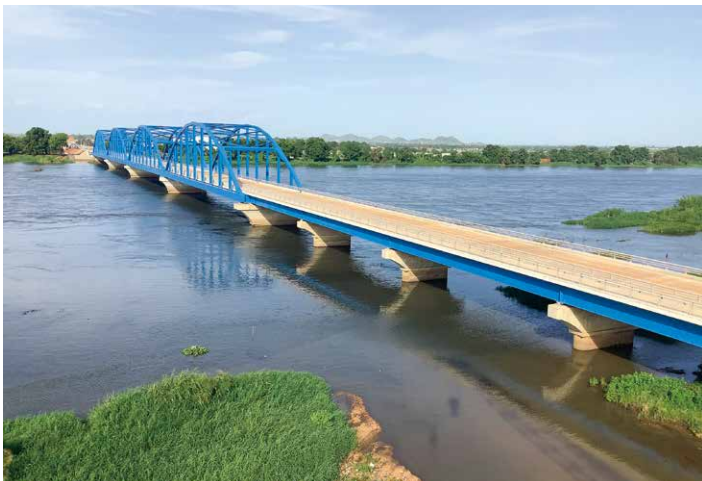
Completed bridge with a long span of 560 m
