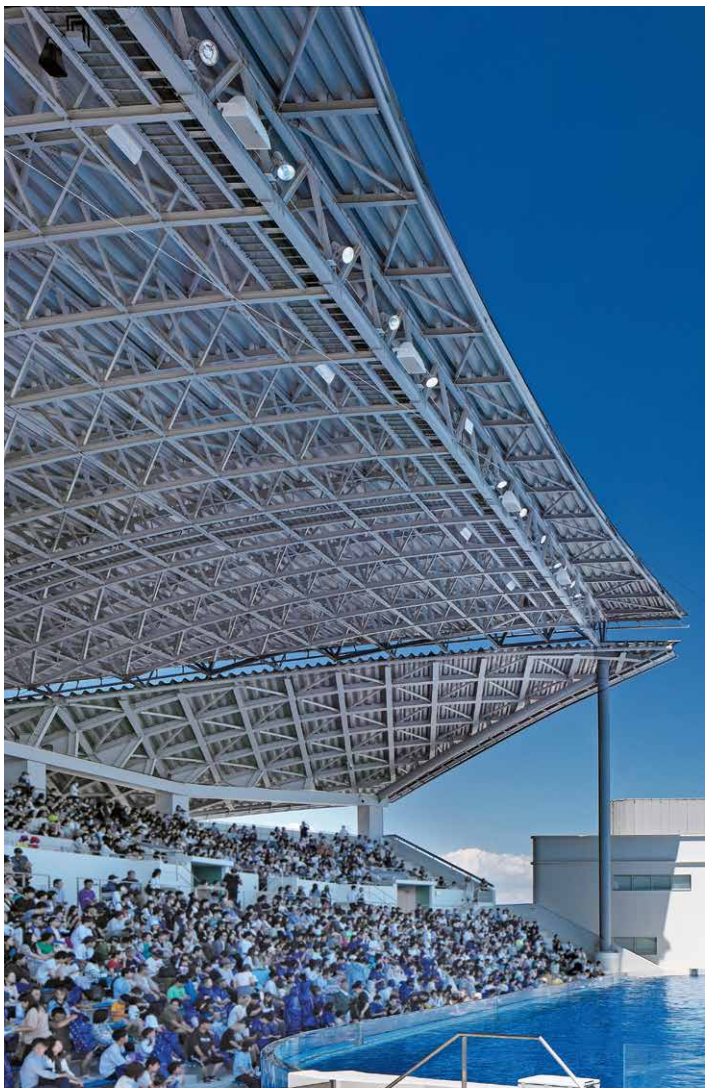
Inside view of the orca stadium (composed of two roofs—upper roof and lower roof)
