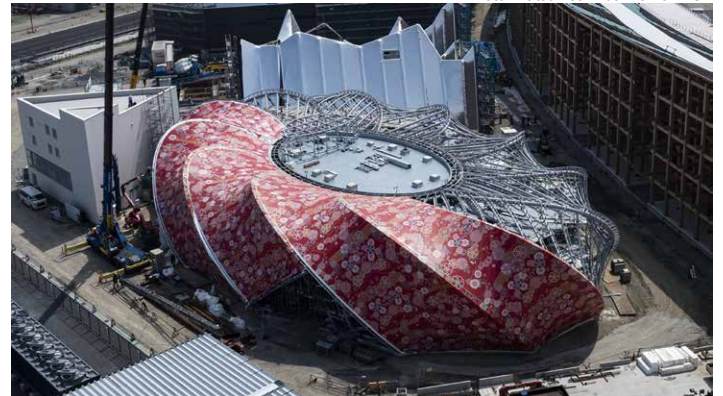
Nishijin-textile membrane erection underway
