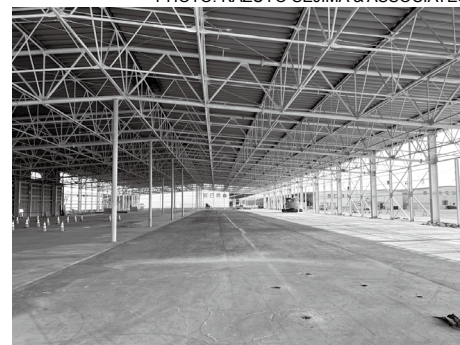
Remodeling of existing factory building: Exterior wall was removed to newly install sashes in the lower section.
