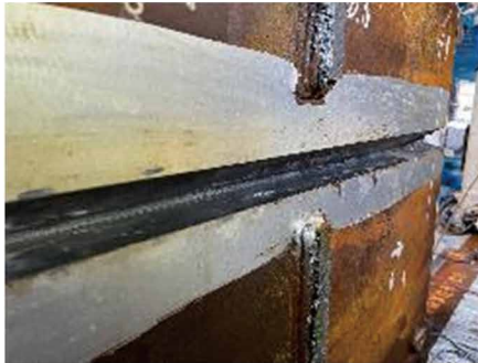
④ Pre-weld groove condition
