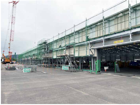
Double-skin exterior wall under construction
