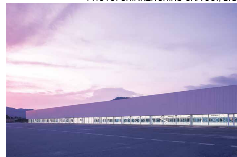
Evening view of the south side of the remodeled factory: Four openings with a height of 2,500 mm were arranged on the lower side of the exterior wall.
