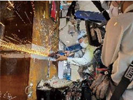
③ Clean weld (protection) removal
