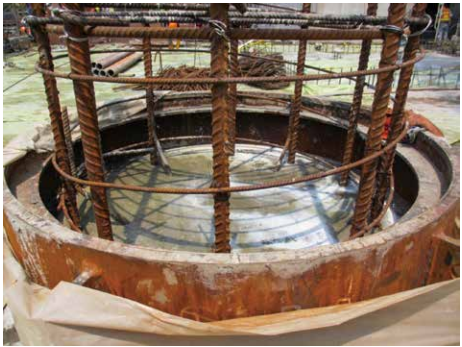
Photo 3 Placement of filling concrete inside CFT column
