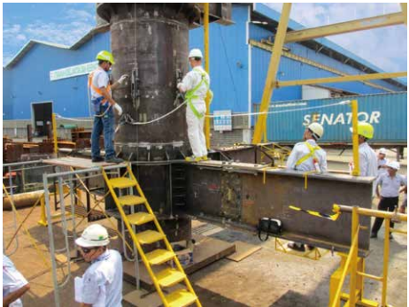
Photo 2 Preparation of mockup of beam-to-column connection at fabrication plant
