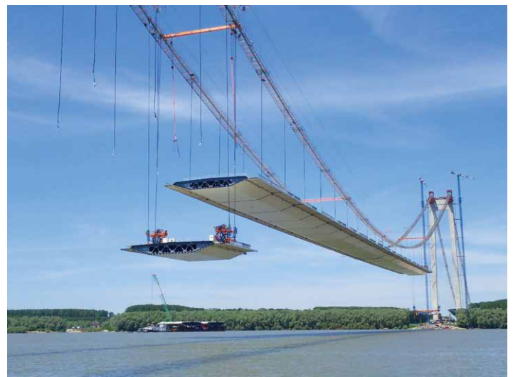
Erection of deck segment
