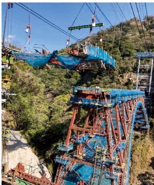
Photo 4 Removal of damaged bridge members
