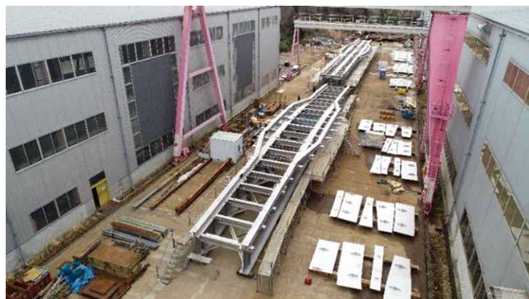
Photo 1 Temporary assembly (front: Tsukishima River Bridge; back Oshima River Bridge)
