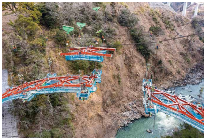
Photo 7 Erection of lower chord members (closing)
