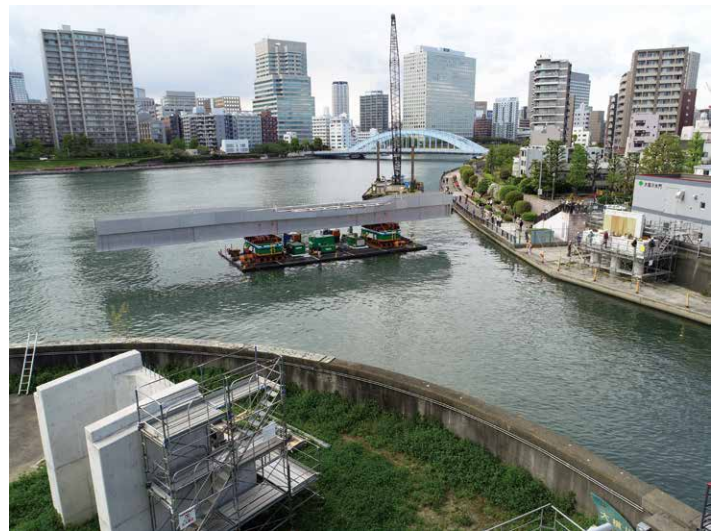
Photo 4 Erection of Oshima River Terrace Connecting Bridge
