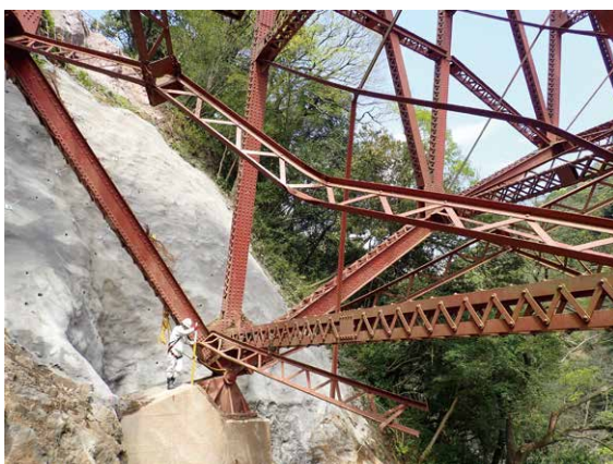
Photo 2 Fracture of sway bracing and lower lateral bracing
