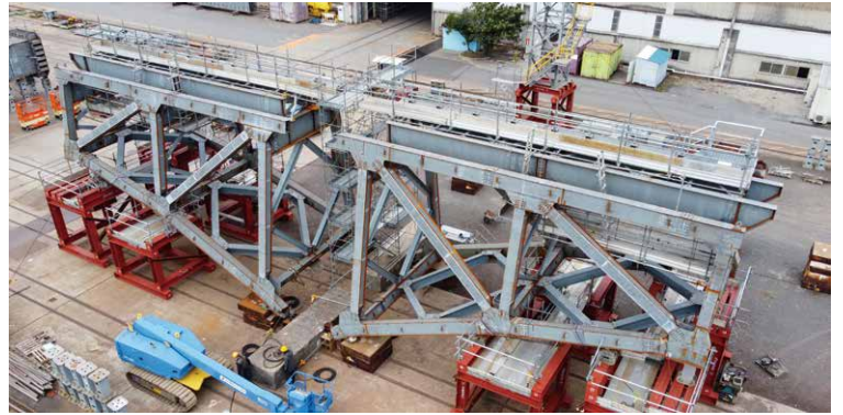
Photo 6 Partial solid temporary assembly
