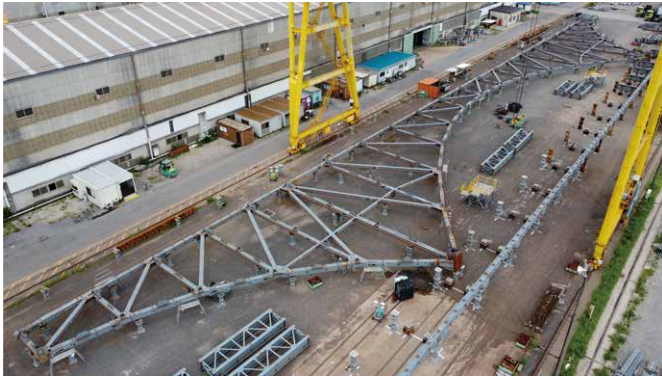
Photo 5 Partial planar temporary assembly
