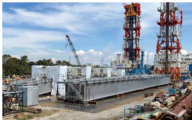
Photo 2 Ground assembly (front: Oshima River Bridge; back: Tsukishima River Bridge)
