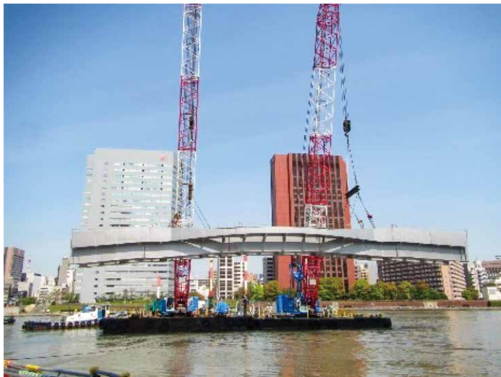
Photo 3 Erection of Tsukishima River Terrace Connecting Bridge
