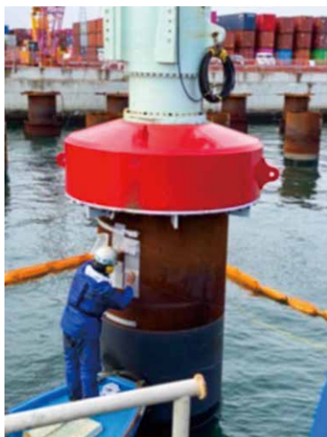
Photo 1 Measurement of penetration and rebound
