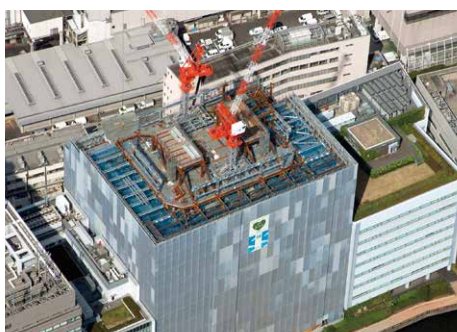
Photo 5 Erection of four trusses to the north and east directions
