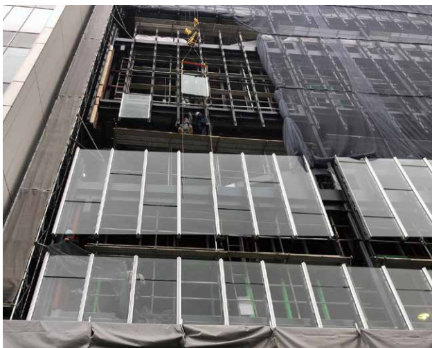
Photo 10 Exterior building construction, with a façade composed of small glass aggregates
