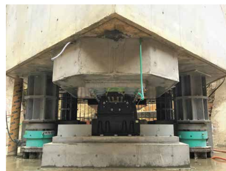
Base-isolation device installed for seismic retrofitting
