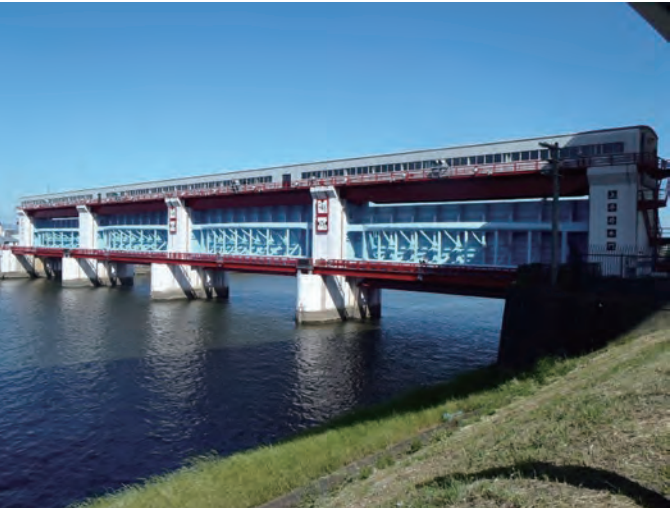
Photo 1 Full view of the flood gate before retrofitting (from upper stream side)
