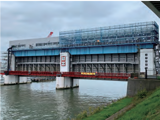
Photo 4 Current on-site condition
