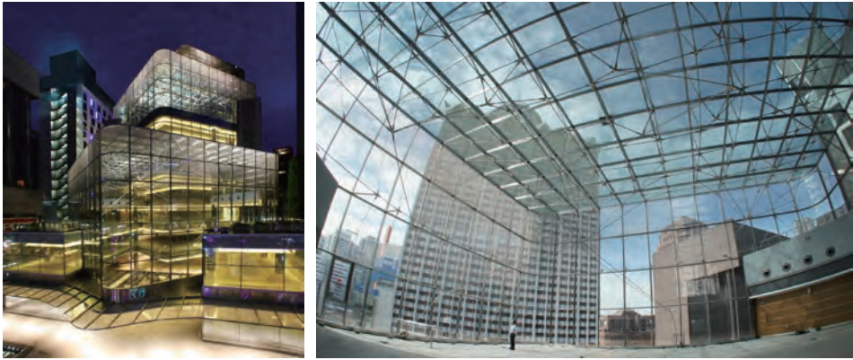
Photo 1 Exterior and interior views
