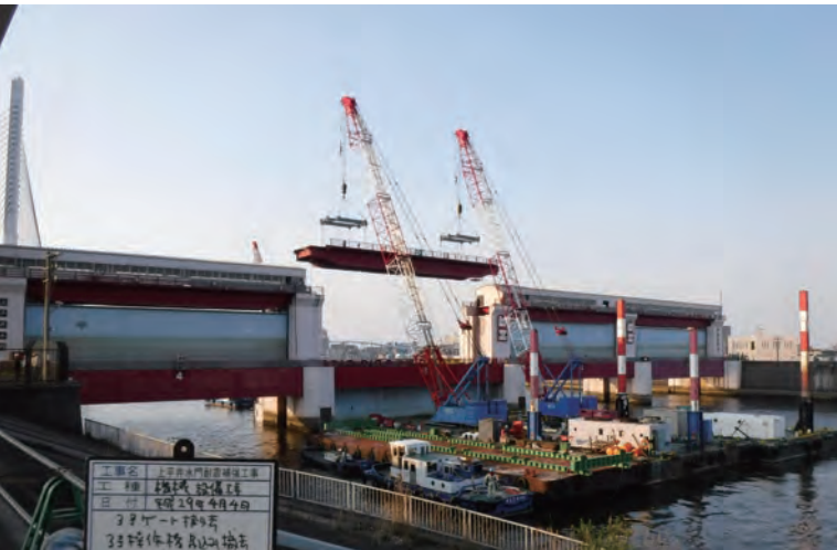
Photo 3 Removal of operation bridge
