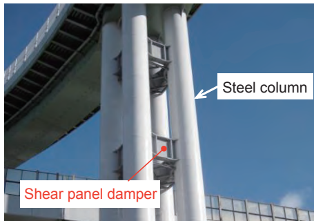
Fig. 1 Multiple Steel Columns
