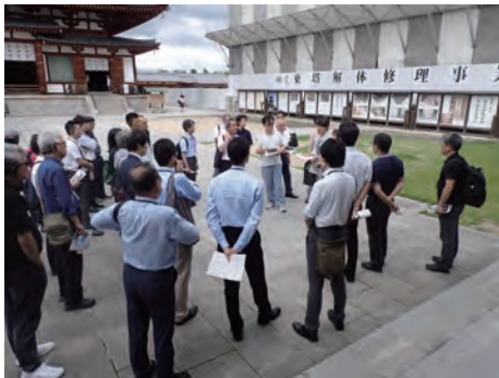
Photo 8 The restoration site of "East Pagoda" in Yakushi-ji Temple
