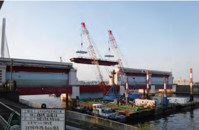
Photo 3 Removal of operation bridge
