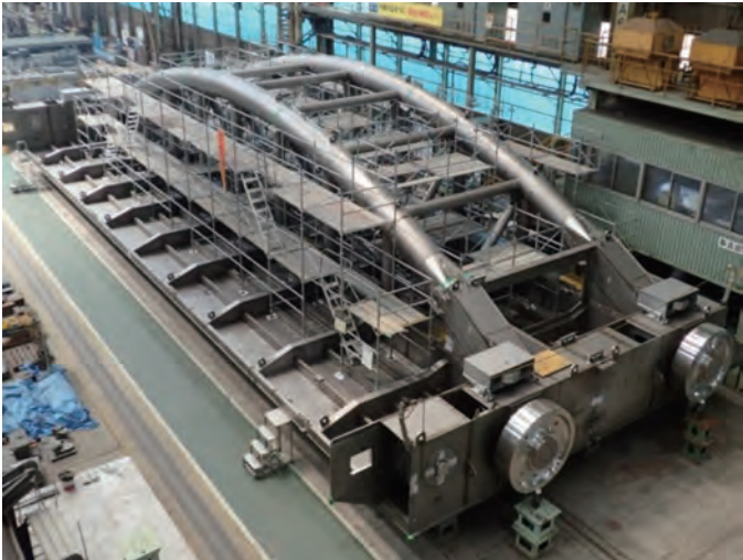
Photo 2 Temporary assembly at fabrication plant
