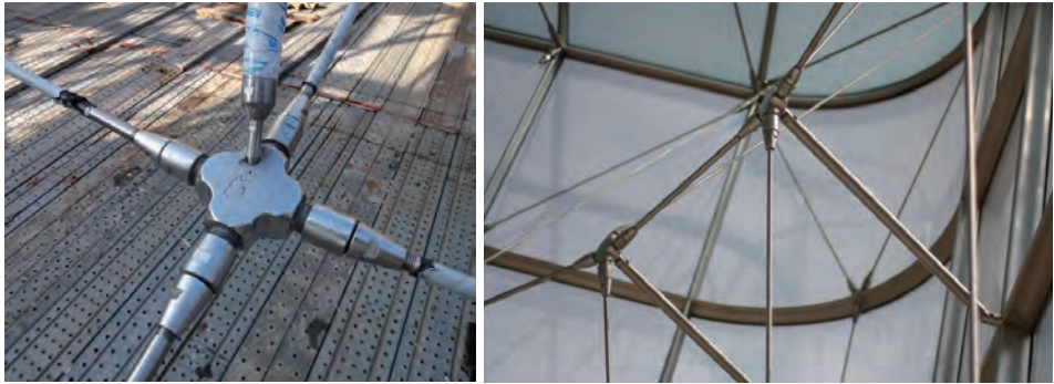
Photo 3 Joint of tension rod
