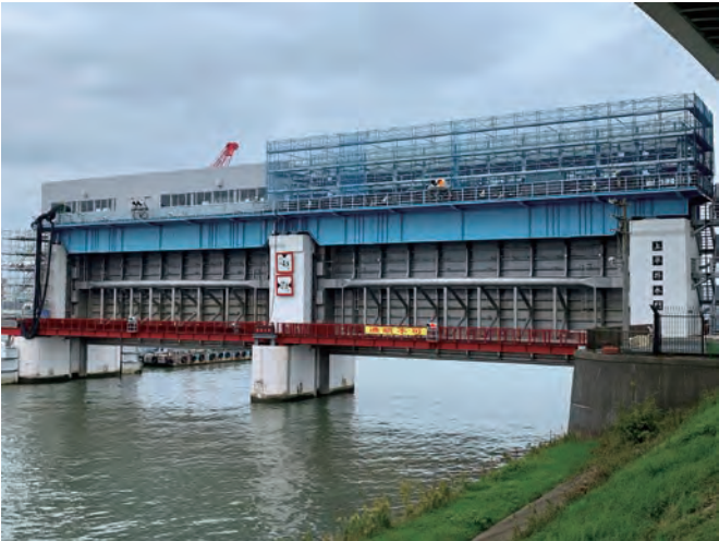
Photo 4 Current on-site condition
