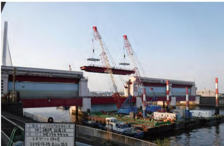
Photo 3 Removal of operation bridge
