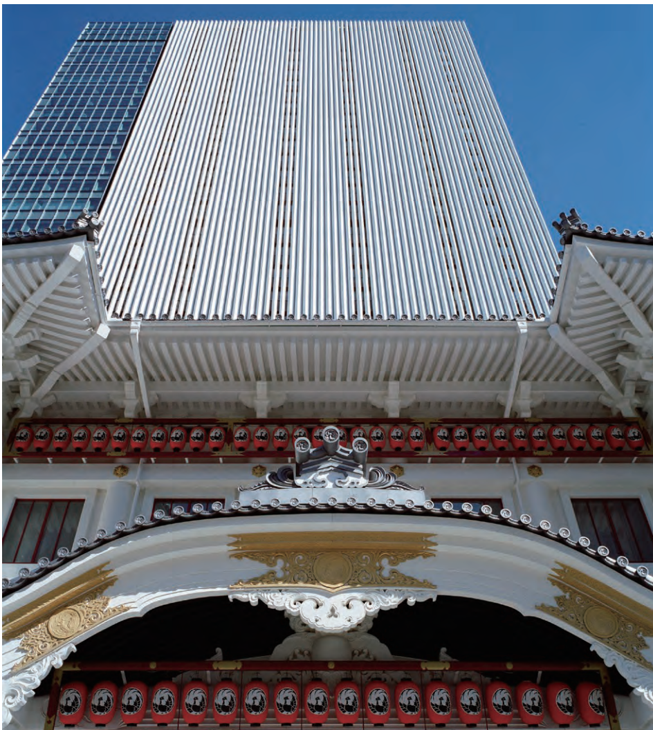
Photo 8 Traditional tile roof of Kabukiza Theatre and vertically-narrow spaced lattice exterior of Kabukiza Building of GINZA KABUKIZA completed by optimized use of steel structure
