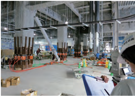
Photo 7 Measurement of displacement of frames during installation
