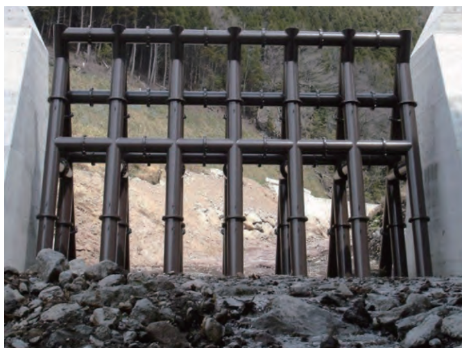
Photo 1 Steel slit dam
