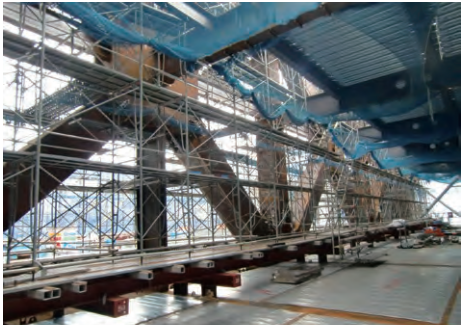
Photo 5 Mega truss with a span of 38.4 m and a height of 13 m and manufactured employing high-strength steel SA440
