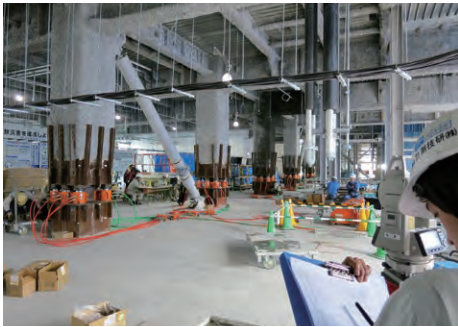
Photo 7 Measurement of displacement of frames during installation
