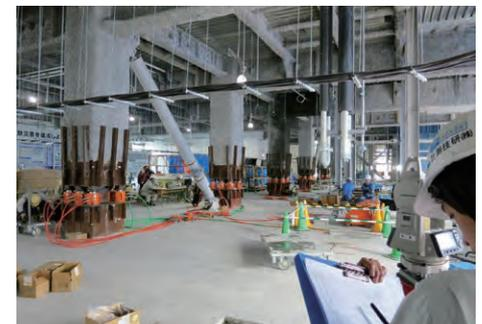
Photo 7 Measurement of displacement of frames during installation
