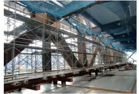
Photo 5 Mega truss with a span of 38.4 m and a height of 13 m and manufactured employing high-strength steel SA440
