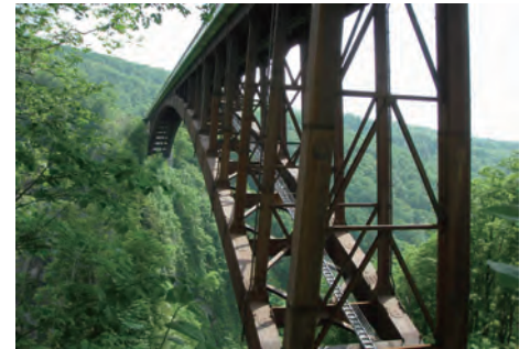
Photo 2 Application of weathering steel bridge in remote mountainous area
