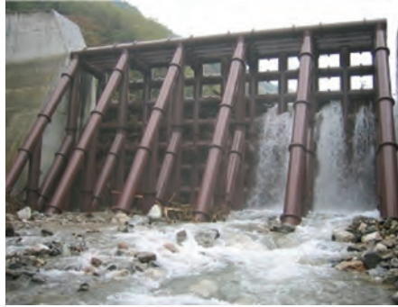
Photo 1 Examples of debris flow-control measures using steel pipes
