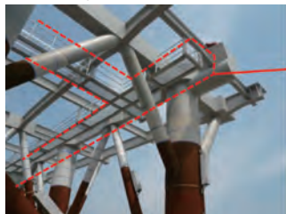
Fig. 3 Example of Design with Consideration to Maintenance Stage (Inspection Catwalk Applied in Jacket-type Wharf)
