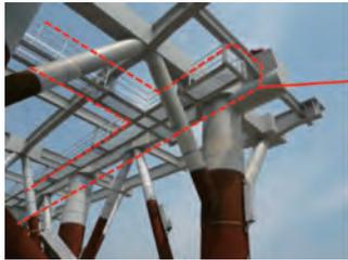
Installation of inspection catwalk from the design stage so as to allow for easy maintenance
