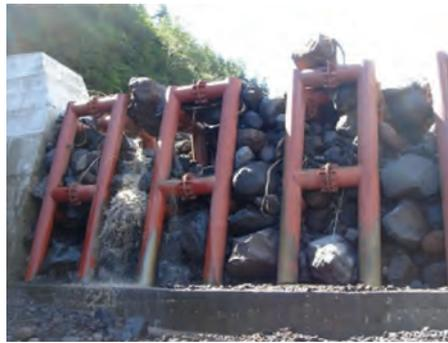
Condition of capturing of debris flow
