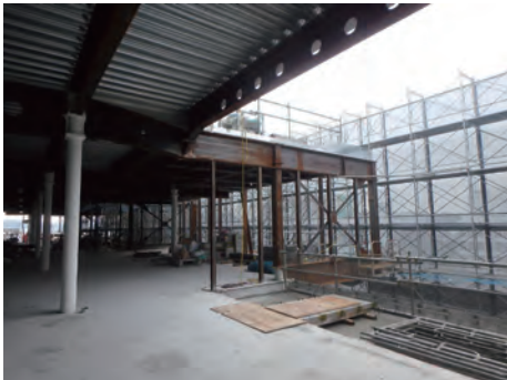
Photo 6 Building structure employing heavy-wall seamless steel tube
