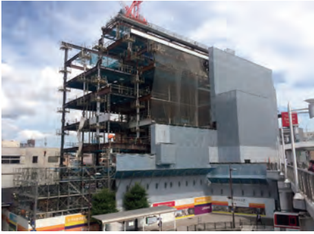
Photo 4 Steel structure construction
