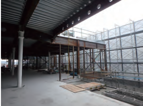
Photo 6 Building structure employing heavy-wall seamless steel tube
