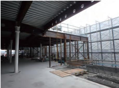
Photo 6 Building structure employing heavy-wall seamless steel tube
