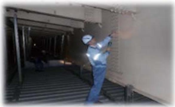
Photo 3 Interior of multi-function corrosion-protection deck
