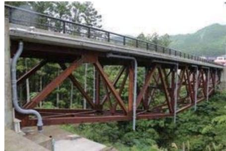
Photo 2 Special-type bridges constructed using weathering steel
