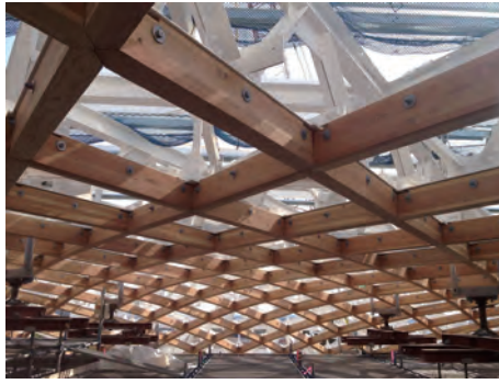
Photo 5 Fixing wood members to lower chord member
