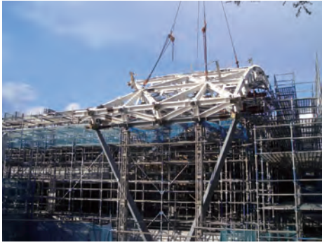
Photo 4 Hoisting and welding of field-assembled roof truss beam units
