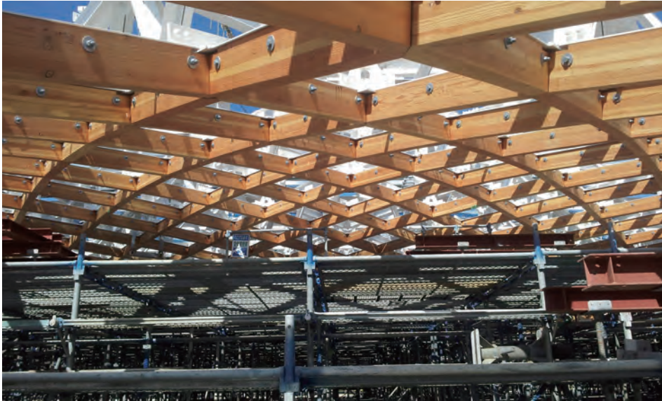
Photo 6 Wood-grid roof structure after jacking down
