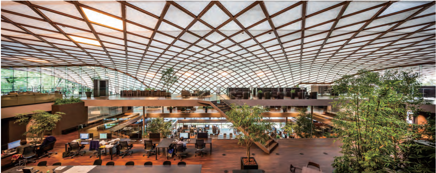
Photo 3 Entire working space seen from 4th floor
