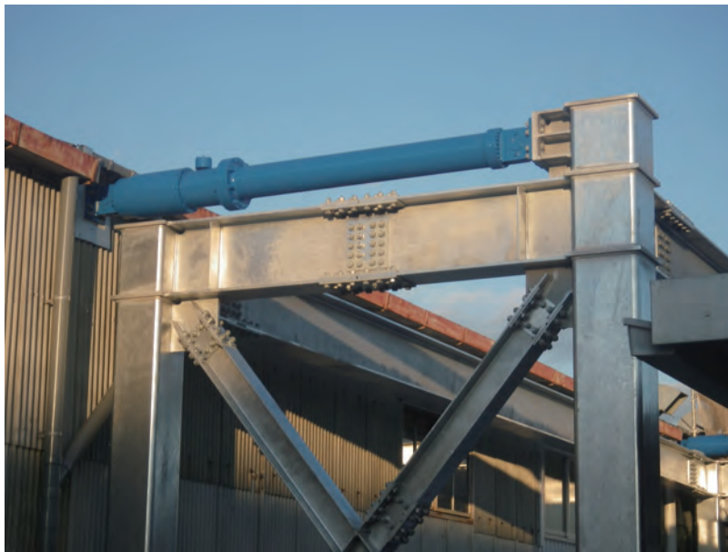
Photo 1 Response-control buttress framing employing viscosity damper
