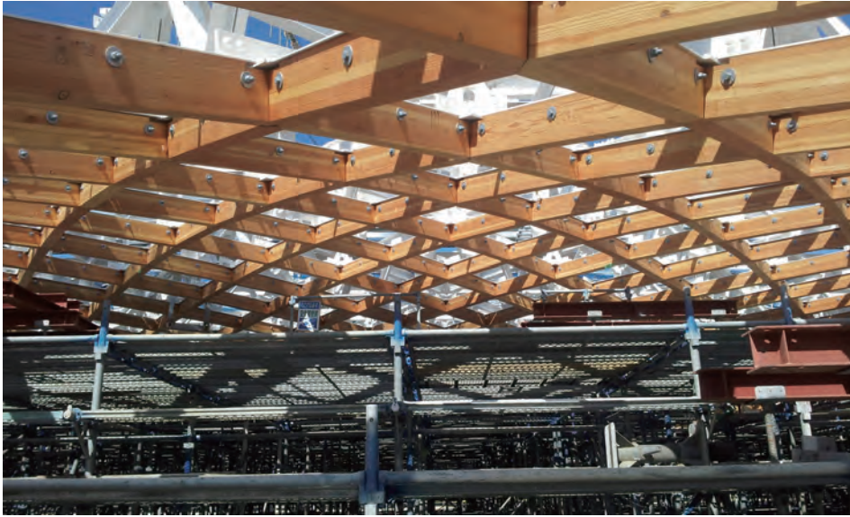
Photo 6 Wood-grid roof structure after jacking down
