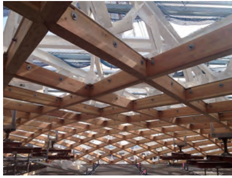
Photo 5 Fixing wood members to lower chord member
