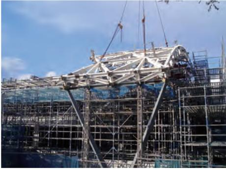
Photo 4 Hoisting and welding of field-assembled roof truss beam units
