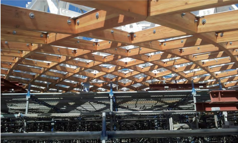
Photo 6 Wood-grid roof structure after jacking down
