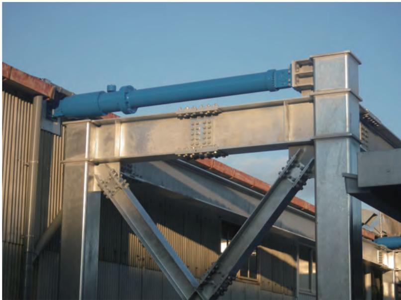
Photo 1 Response-control buttress framing employing viscosity damper
