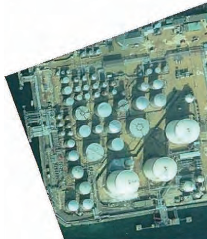
(a) Soil liquefaction (The yellow colored ground surface shows the thick deposit by the boiling of liquefied sand)
