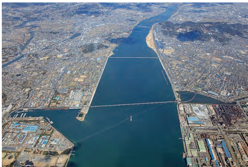
Photo 3 The Kurashiki Minato Bridge under construction at the testing site was completed and opened to traffic in March 2017 (foreground)
