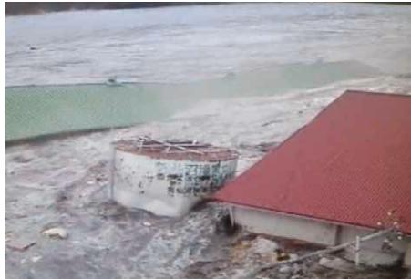
Photo 4 Floating out of oil tanks into the sea by the tsunami (2011 East Japan earthquake)
