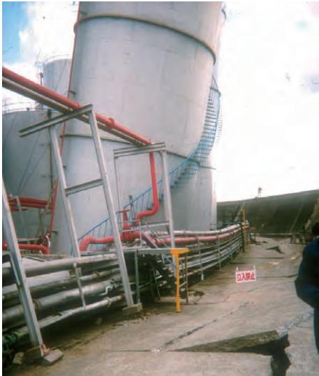
Photo 3 Settlement and inclination of oil product tank by soil liquefaction (1995 Kobe earthquake)
