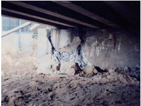
Photo 1 Damage to bridge abutment located in the ground where liquefaction occurred<sup>2)</sup>
