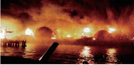
Photo 1 Explosion and fire of 17 spherical LPG tanks (2011 East Japan earthquake)
