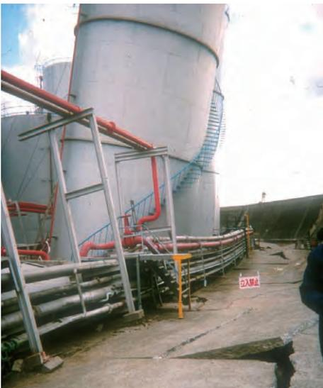
Photo 3 Settlement and inclination of oil product tank by soil liquefaction (1995 Kobe earthquake)
