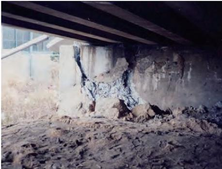
Photo 1 Damage to bridge abutment located in the ground where liquefaction occurred<sup>2)</sup>
