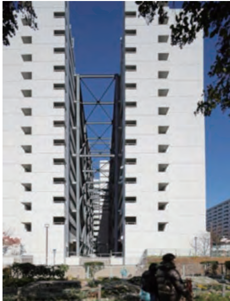
Photo 1 Kawaramachi housing after seismic retrofitting
