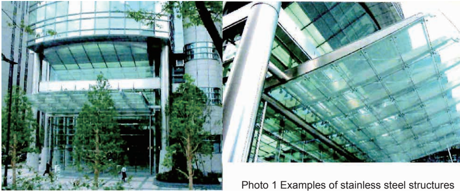
Photo 1 Examples of stainless steel structures
