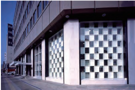
Photo 1 Appearance of the building (after retrofitting)
