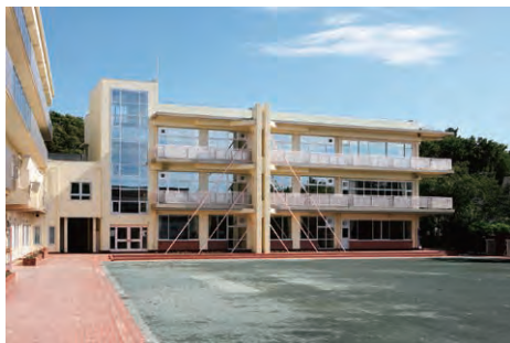
Photo 1 Appearance of East School Building after seismic retrofitting by means of Parallel Structural Method
