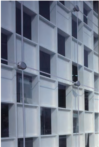
Photo 3 Details of façade
