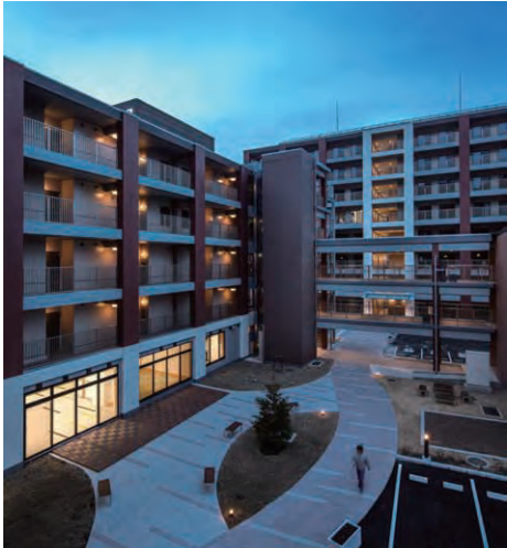
Photo 1 Appearance seen from courtyard
