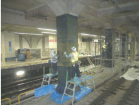
Photo 3 Seismic retrofitting of platform columns by means of carbon fiber wrapping
