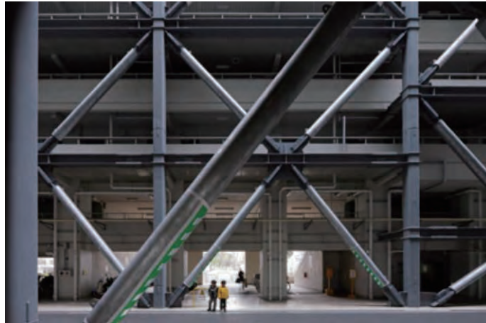
Photo 2 "Skip arrangement" of mega response-control frame
