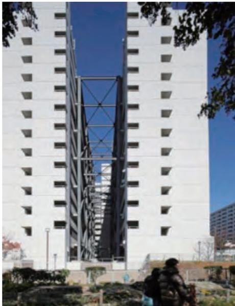
Photo 1 Kawaramachi housing after seismic retrofitting
