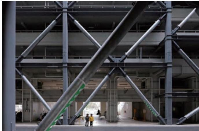
Photo 2 "Skip arrangement" of mega response-control frame
