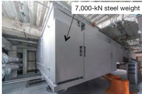
Photo 1 Appearance of "Dual TMD-NT"
