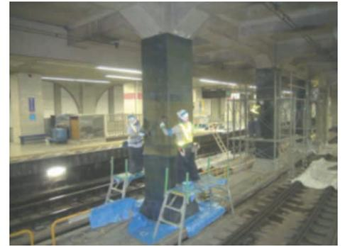
Photo 3 Seismic retrofitting of platform columns by means of carbon fiber wrapping
