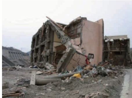
Photo 3 Building that overturned due to tsunamis
