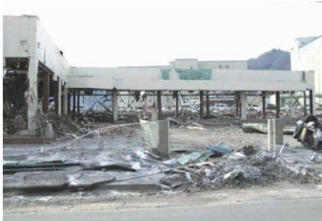
While exterior members were washed out and fracture of brace was found, the building structure remained intact.
