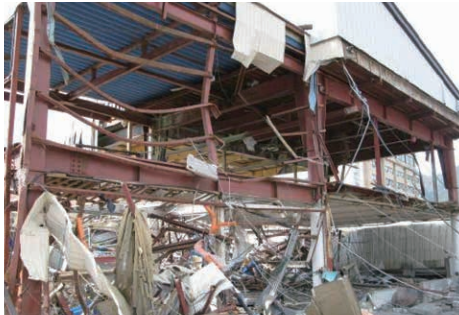
While studs caused deformation due to collision of drifts, the building framing remained intact.
