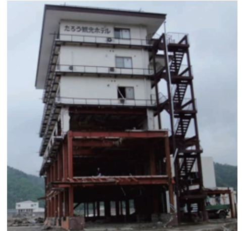
Photo 5 Steel-structure building where exterior and interior members were washed away by tsunamis
