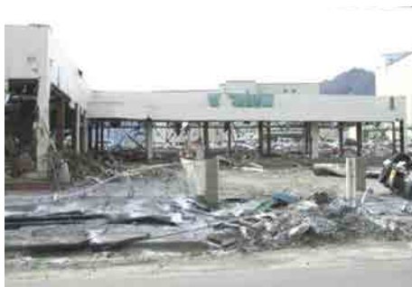
While exterior members were washed out and fracture of brace was found, the building structure remained intact.
