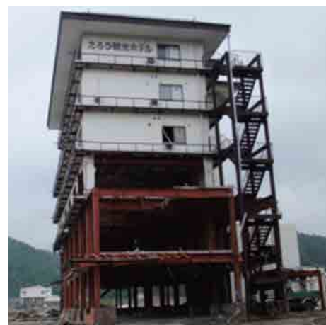
Photo 5 Steel-structure building where exterior and interior members were washed away by tsunamis
