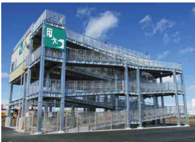
Photo 4 Two-story steel structure Nakano 5-chome Tsunami Evacuation Tower developed and constructed in Sendai City
