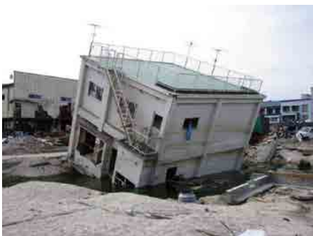
Photo 4 Building that inclined due to scouring
