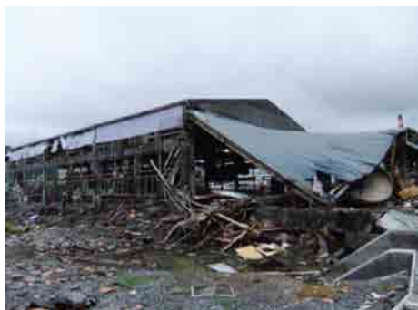
Photo 2 Steel-structure building with which drifts (ship) collided
