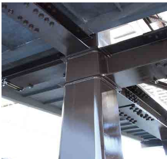
Steel tube column-H-shape structure in which square steel tube is used for column and H-shape for beam
