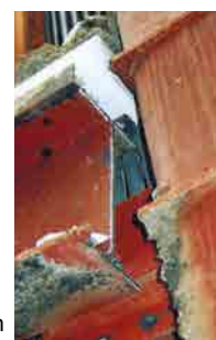
Fracture at beam end that occurred prior to its sufficient deformation
