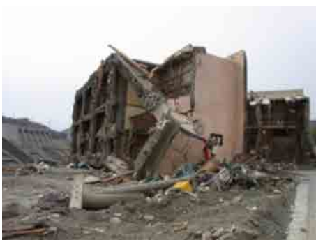
Photo 3 Building that overturned due to tsunamis
