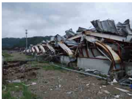
Photo 1 Steel-structure building destroyed by tsunamis
