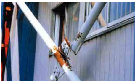
Fracture of brace connection
