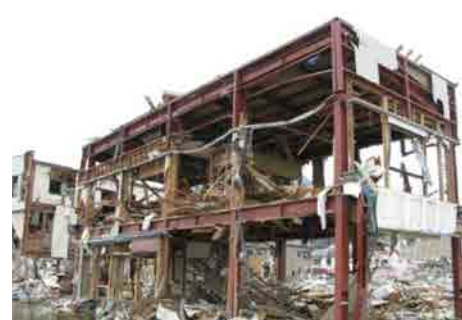
While exterior members were washed out, the building framing remained intact.
