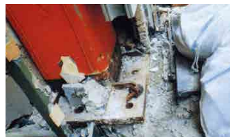
Fracture of anchor bolts of column base to cause dislocation of column
