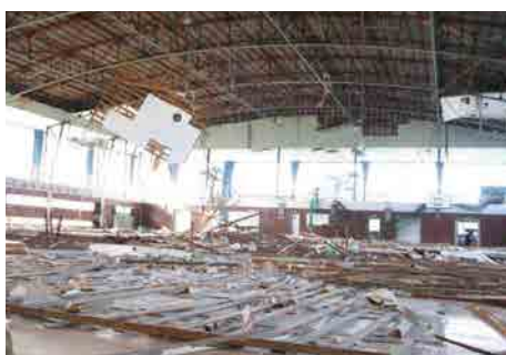
Ceiling members fell due to earthquakes.
