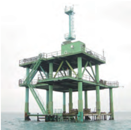
Photo 1 Full view of Marine Engineering Research Facility
