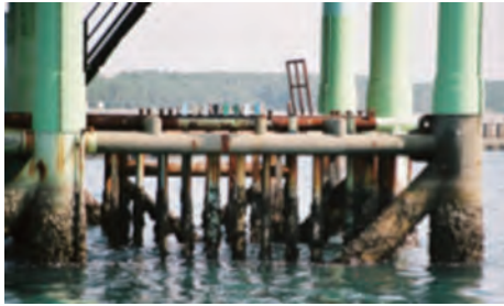
Photo 1 Exposure test conditions
