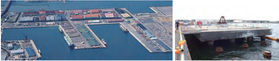
Photo 1 Overview of Shiomi Wharf No.3 of Sakai-Senboku Port (Osaka Prefecture, Port Authority)
