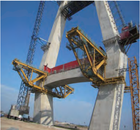
Photo 1 View of construction by inclined bent
