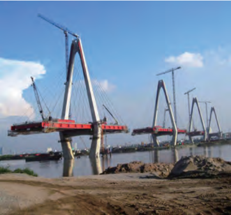
Photo 2 View of construction by cantilever erection
