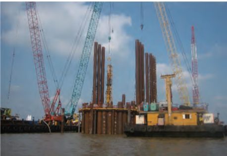
Photo 3 SPSP installation
