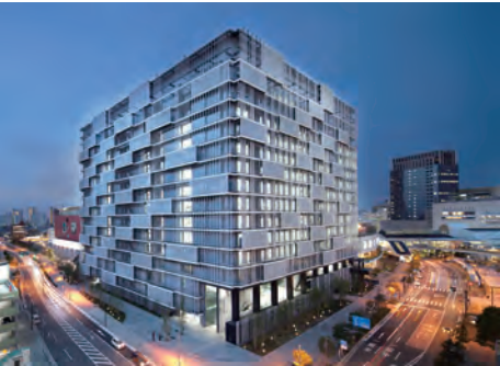
Photo 1 Lazona Kawasaki Toshiba Building
