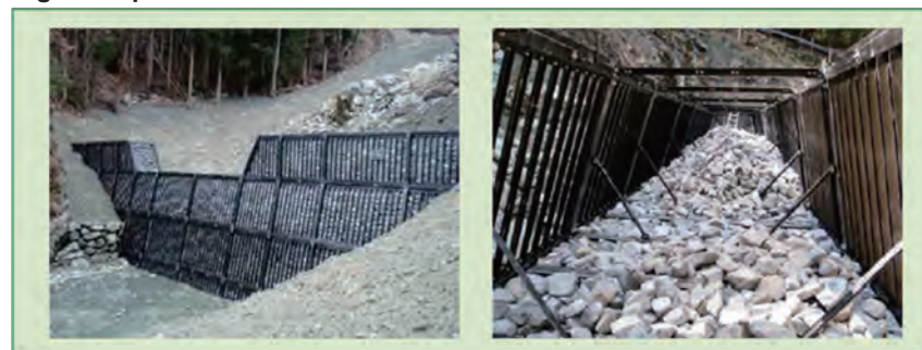
Fig. 11 Impermeable Steel Dam to Block Sand
