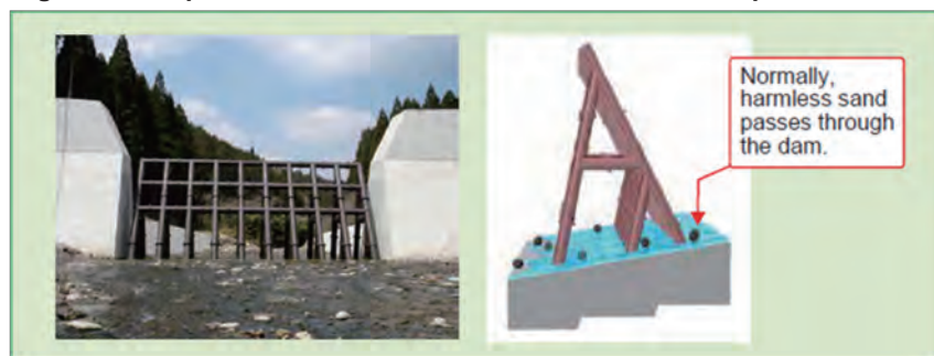
Fig. 10 Water-permeable Steel Dam to Prevent Sand Buildup
