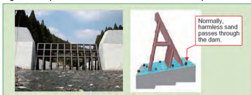
Fig. 10 Water-permeable Steel Dam to Prevent Sand Buildup
