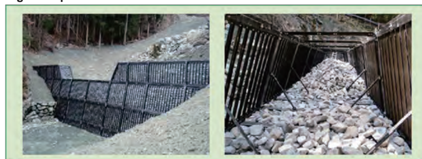
Fig. 11 Impermeable Steel Dam to Block Sand
