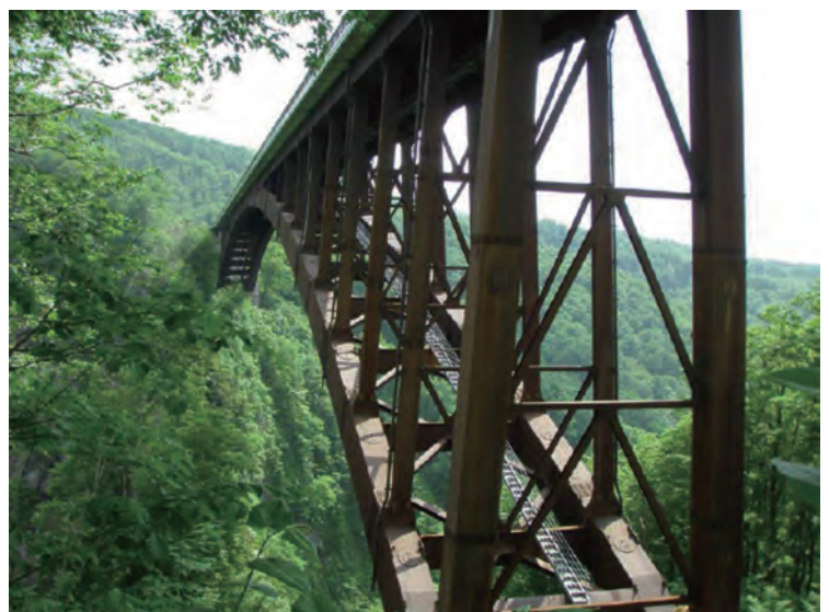
Application of weathering steel bridge in remote mountainous area
