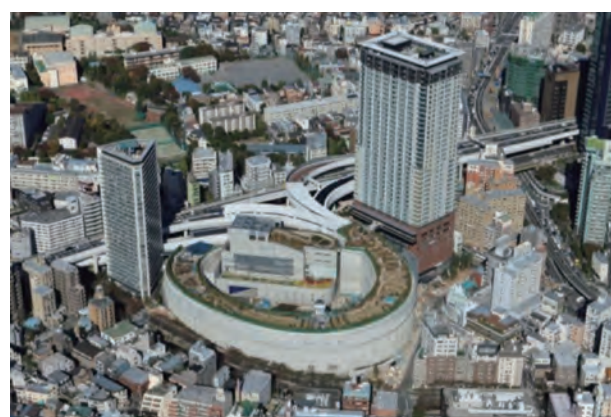
Photo 1 Full view of Ohashi Junction
