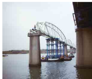
Simultaneous bridge dismantling method using barge
