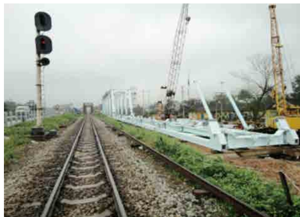
Photo 1 Yard assembly of new bridge at No. 20 Truoi Bridge site
