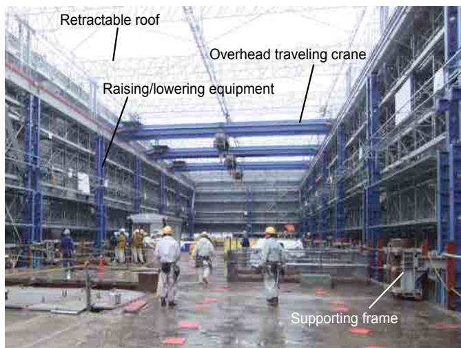
Photo 3 Demolition equipment in hat
