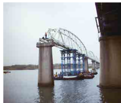
Photo 3 Simultaneous dismantling method for whole bridge structures using barge
