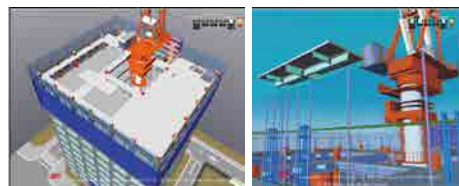
Fig. 1 Verification of Demolition Process Employing 3-dimensional Image (removal of slab)
