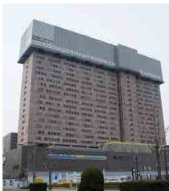
Upper-floor closure-type demolition method
