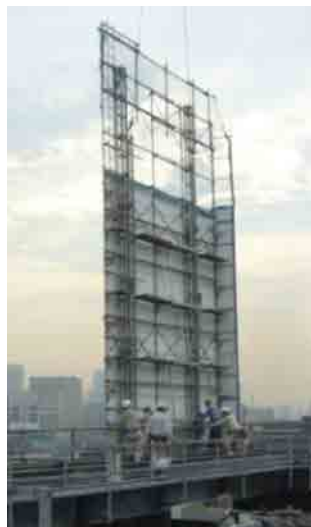
Photo 5 A piece of movable peripheral protection unit scaffolding system (assembly into 2 units in a lump)
