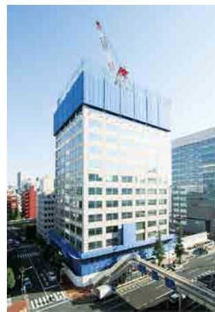
Reverse construction demolition method
