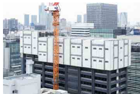
Photo 2 Demolition using Cube Cut method
