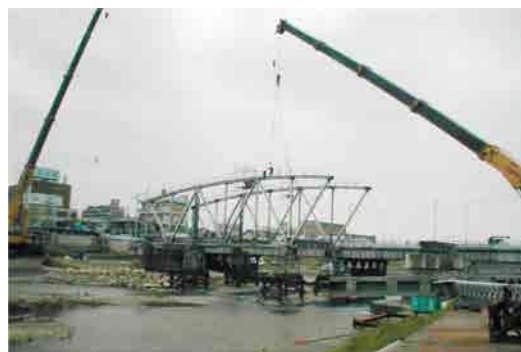
Photo 1 Bent method using truck crane (block dismantling)
