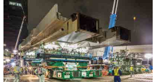
Photo 2 Upper: Girder replacing condition Lower: Girder removal and transport
