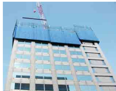
Photo 4 Moving down of peripheral protection unit scaffolding for use for lower floor (moving down of 2 units in a lump)
