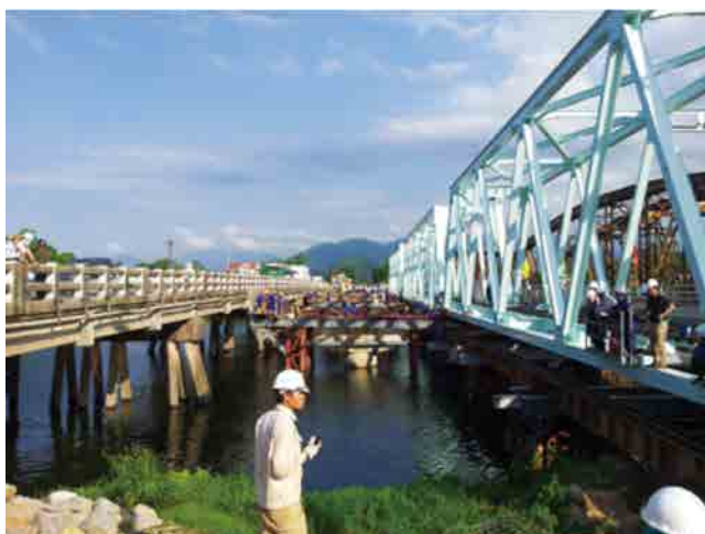
Photo 3 Lateral transfer of new bridge at No. 20 Truoi Bridge
