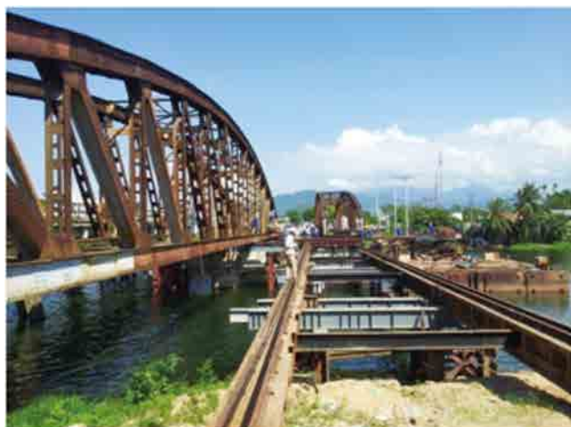
Photo 2 Lateral transfer of existing bridge at No. 20 Truoi Bridge site
