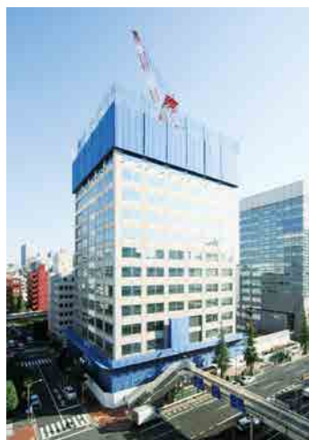
Photo 1 SHIMIZU Reverse Construction Demolition Method underway
