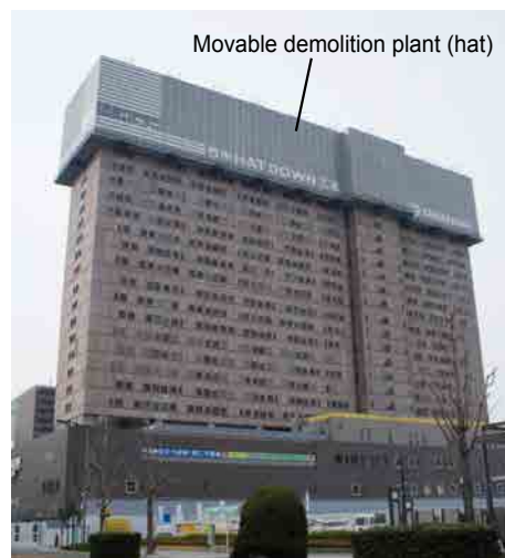
Photo 2 Full view of movable demolition plant (hat)
