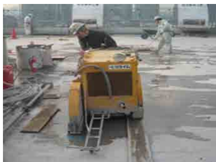
Photo 3 Cutting of slab
