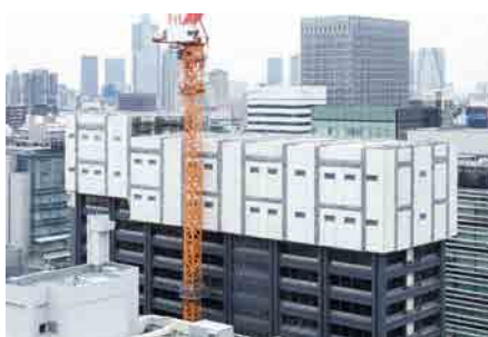
Cube cut demolition method
