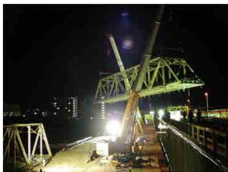
Photo 2 Simultaneous dismantling method for whole bridge structures using crane
