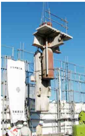
Photo 2 Cut and removal of concrete-filled steel tube column
