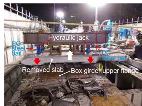
Photo 1 Concrete slab removal by means of jack-up method
