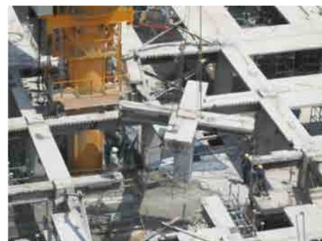
Photo 1 Removal of columns and beams
