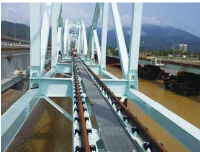
Photo 4 Direct rail fastening system for directly laid railway
