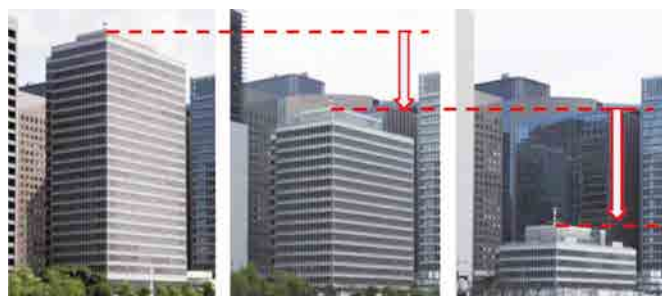
Photo 1 Full view of demolition employing cut and take down method
