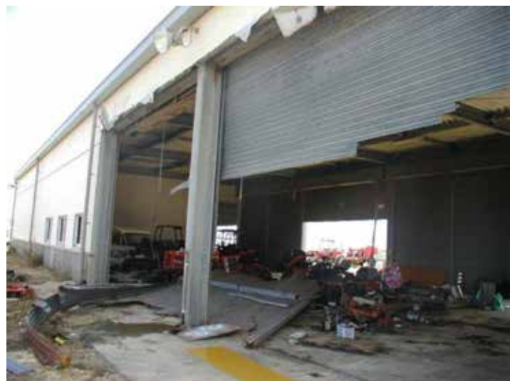
Photo 3 Example of damage caused by typhoon (Miyakojima, Okinawa in 2003)
