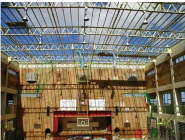
Photo 2 Example of damage caused by typhoon (Miyakojima, Okinawa in 2003)
