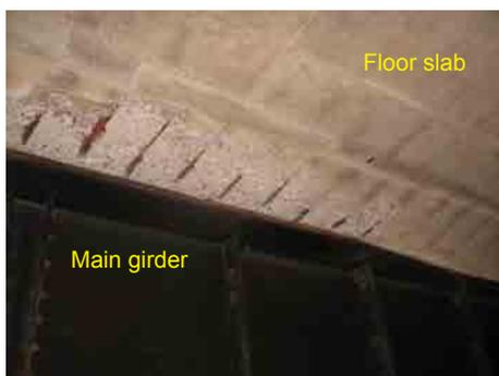
Photo 2 Exposure of steel reinforcement of RC slab (photo taken in 2006)
