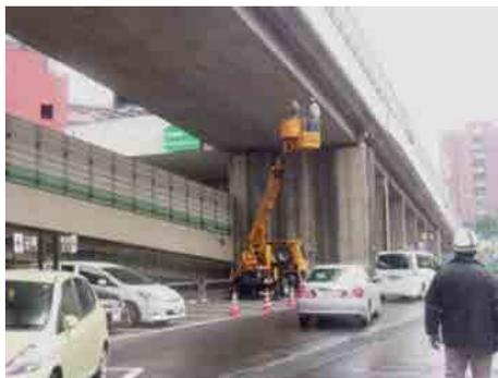
Photo 3 Close-range inspection (inspection by cherry picker; daytime inspection is available at sites where traffic flow is not adversely affected)
