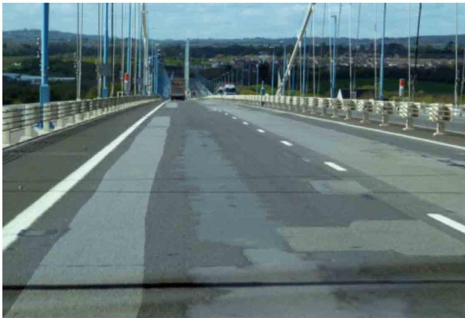
Photo 2 Condition of surfacing at Severn Bridge
