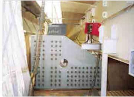
Photo 6 Reinforcement of steel bridge pier by splicing steel plate to pier
