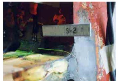
Photo 5 Occurrence of fatigue cracking (observed in weld line where beam and column cross)
