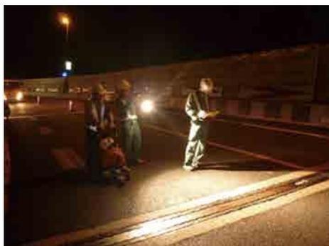
Photo 2 Walking inspection (walking inspection of structures by inspectors in areas of restricted traffic flow during nighttime)
