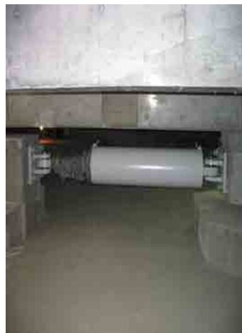
Photo 4 Advanced base-isolation systems (base-isolation laminated rubber and oil damper) were adopted for securing sufficient seismic resistance of the renewed Tokyo Station Building.
