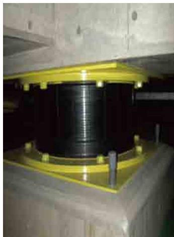
Photo 4 Advanced base-isolation systems (base-isolation laminated rubber and oil damper) were adopted for securing sufficient seismic resistance of the renewed Tokyo Station Building.
