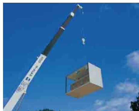
Photo 17 Installation of unit structure
