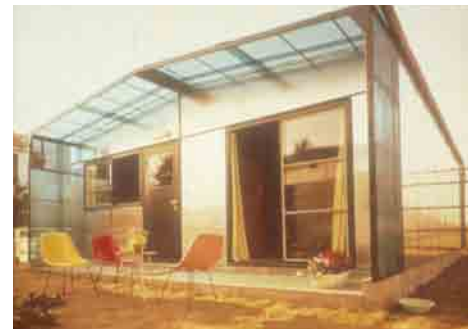
Photo 1 A prefabricated steel-frame house in the initial day and marketed in 1960. Brilliant aluminum wall, new steel sash, and plastic-made eaves and buttress were impressive.
