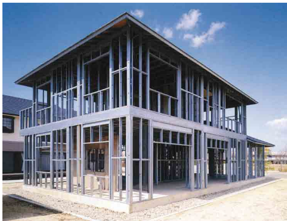
Photo 2 Framing of steel-framed house employing light-gauge steel shapes
