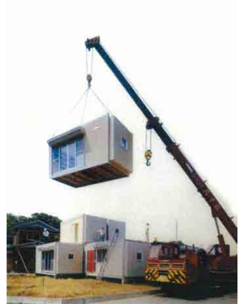
Photo 12 Installation of unit structure
