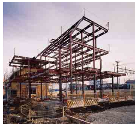
Photo 5 Example of 3-story house employing heavyweight rigid steel frame system
