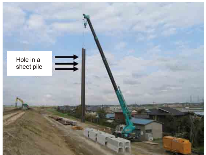
Photo 4 Reconstruction of land side of Tone River levee at Sakae by installing sheet pile walls with holes
