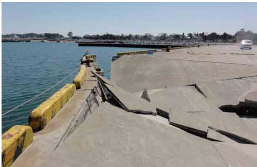
Photo 3 Damage to the steel sheet pile quay wall edge portion in Soma Port during the 2011 Off the Pacific coast of Tohoku Earthquake
