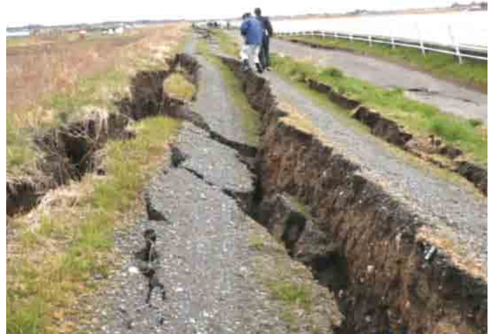
Photo 2 Significant distortion of the Hinuma levee
