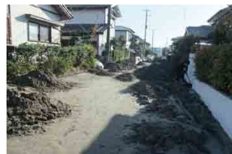
Photo 4 Thick boiled soil observed in Chiba City
