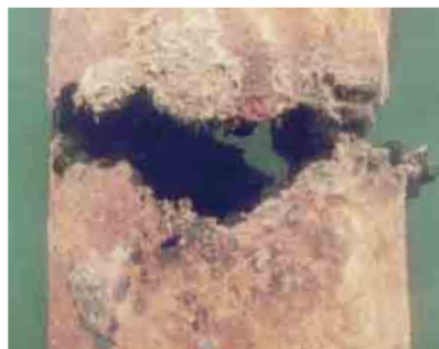
Photo 1 Local corrosion that occurred in port structures: steel sheet pile (left) and steel pipe pile (right)
