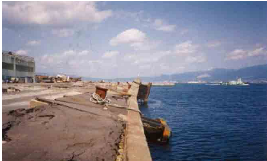
Photo 1 Damage to the steel sheet pile quay wall of Hakodate Port during the 1993 Hokkaido-Nansei-Oki Earthquake
