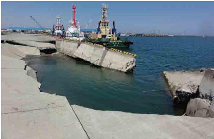
Photo 2 Damage to the steel sheet pile quay wall of Soma Port during the 2011 Off the Pacific coast of Tohoku Earthquake
