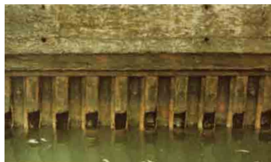
Photo 1 Local corrosion that occurred in port structures: steel sheet pile (left) and steel pipe pile (right)
