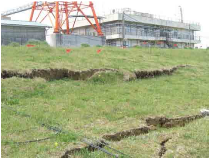
Photo 1 Significant distortion of levee of Tone River in Sawara
