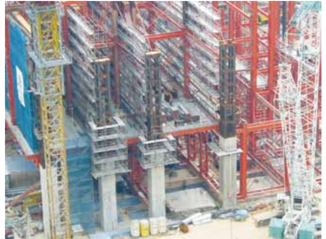
Photo 3 Mega column construction
