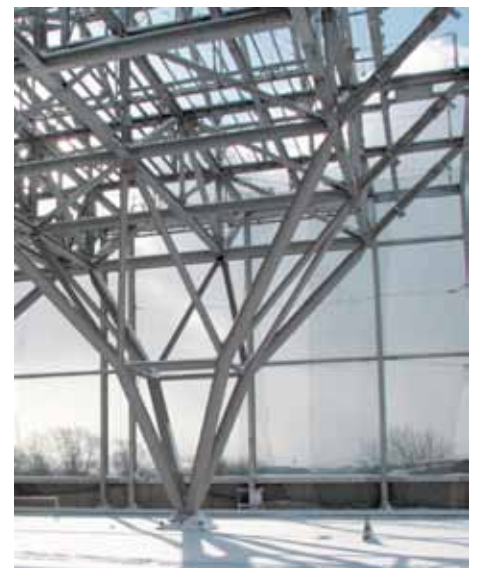
Photo 4 Completed four-branched tubular steel column
