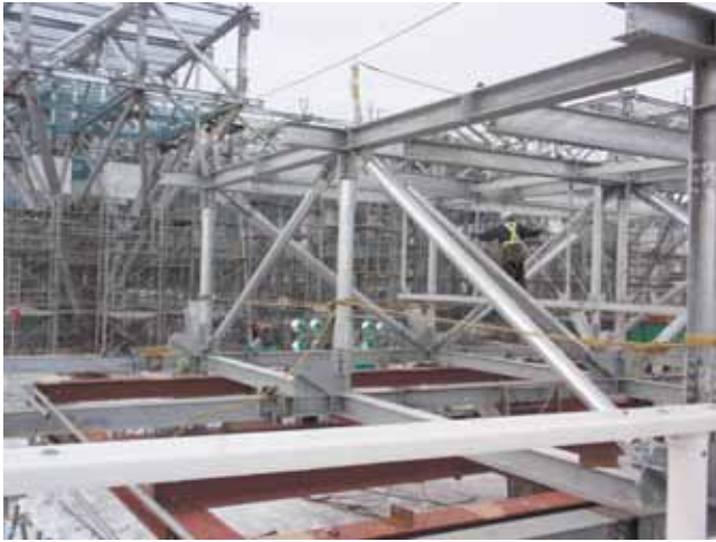
Photo 3 Roof framing
