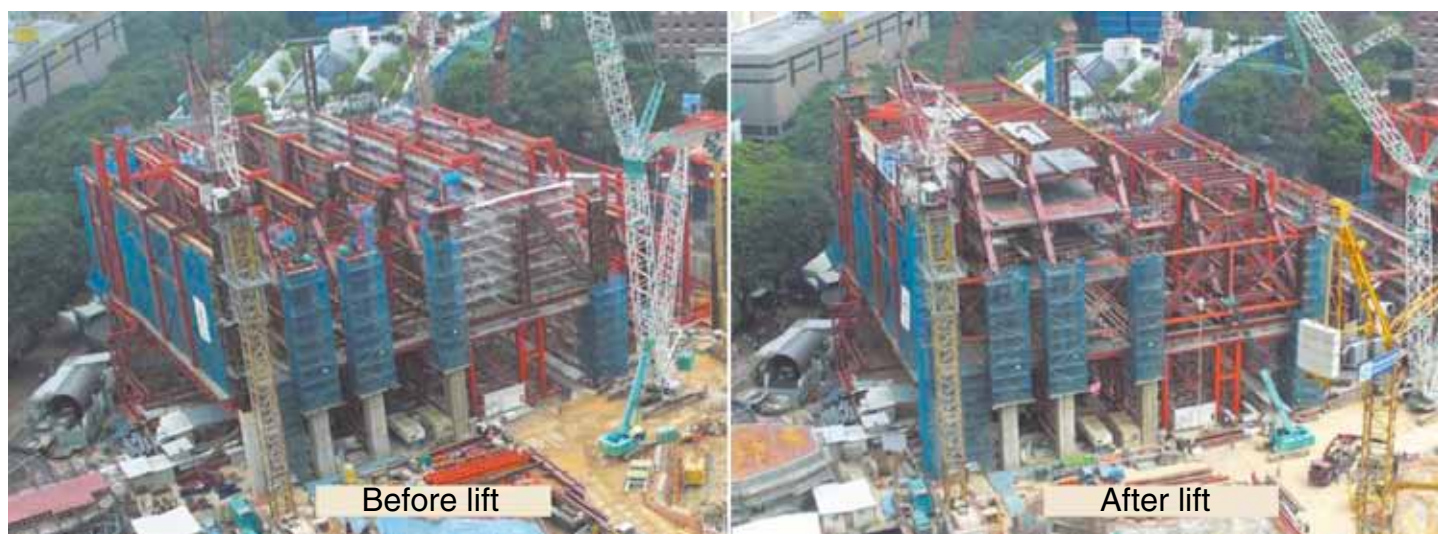
Photo 5 Mega truss work before and after lifting
