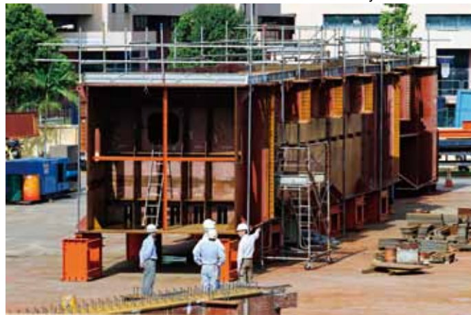
Photo 4 Trial assembly at Yongnam E&C
