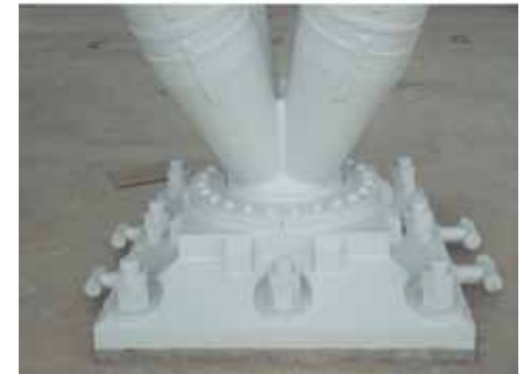
Photo 5 Cast steel pin bearing
