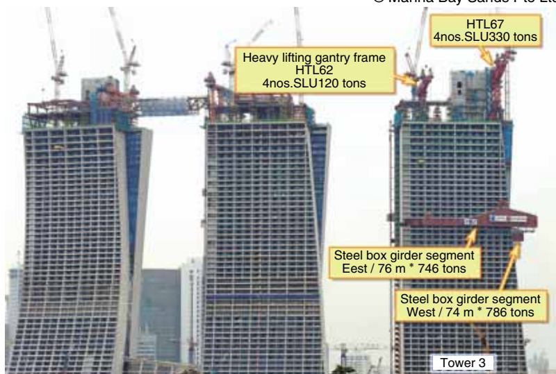
Photo 7 Heavy lifting of box girder bridge segment at Tower 3
