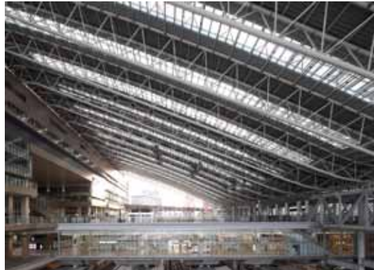
Photo 2 Large-scale domed roof on the station building on the passageway bridge
