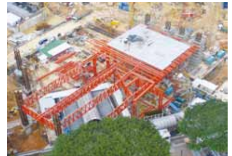
Photo 4 Mega truss assembly (temporary platform)
