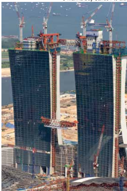
Photo 5 Heavy lifting of steel truss bridge segment
