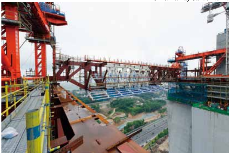
Photo 6 Sliding of steel truss bridge segment into the specified position
