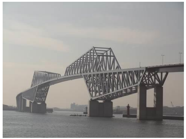
Tokyo Gate Bridge
