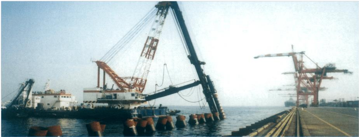
The third berth of Tokyo Ooi container wharf
