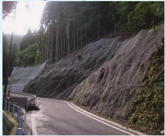
2. Falling-stone protection net
