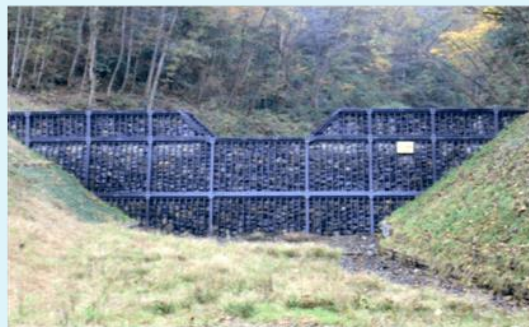
Mountain stream erosion prevention
