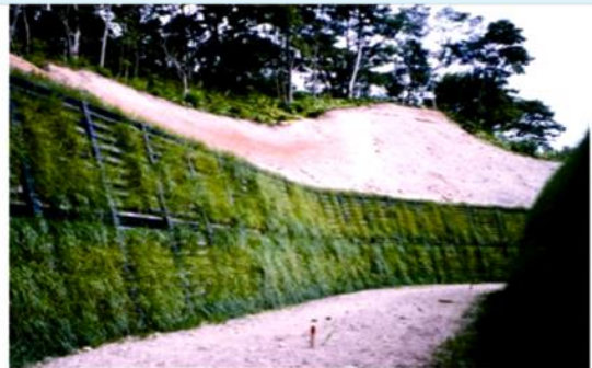
Soil retention work (surface greenery planting)
