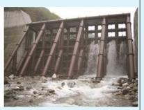
Slit-type structure is designed considering the ecosystem, which does not disrupt river flow
